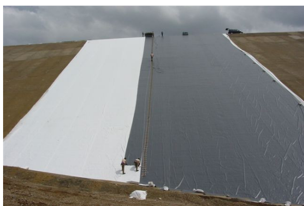
Application of 1st geotextile and ALKORPLAN 35053
